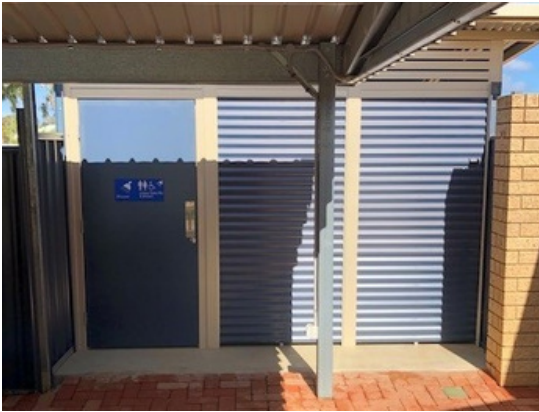
Images: Accessible Toilet at the Boddington Swimming Pool
