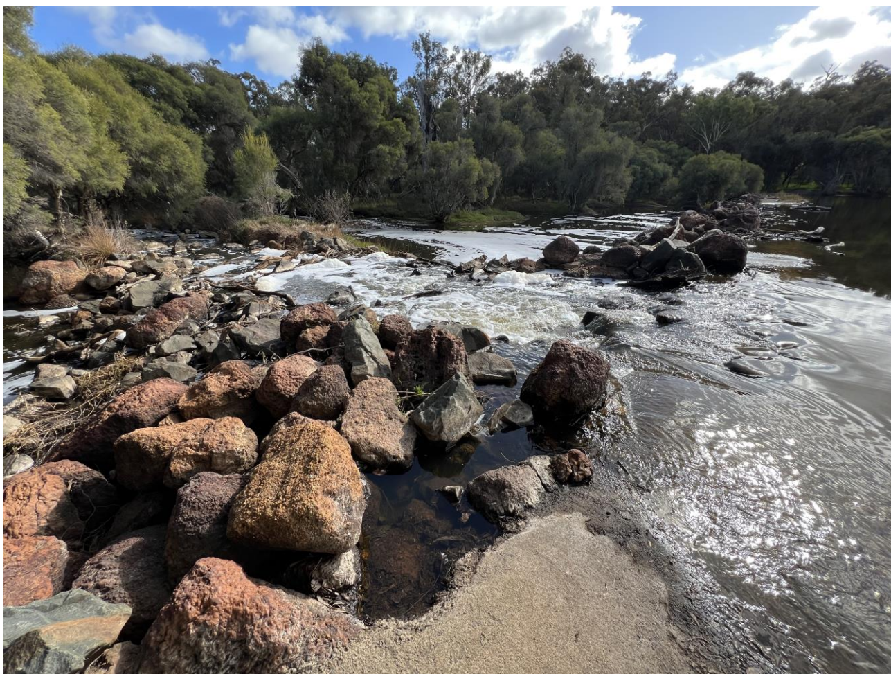
Figure 4:Photo of Fish Ladder and Weir.
