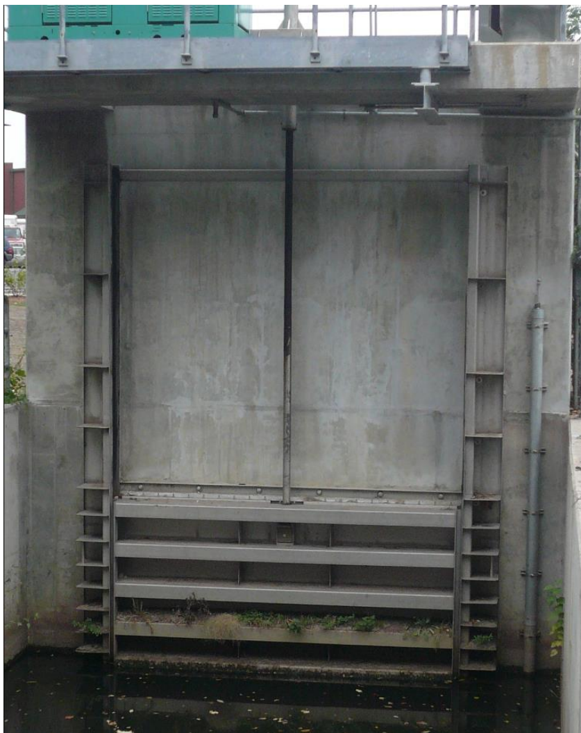
Figure 8: Photo of a sluice gate.
