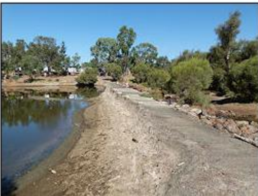
Figure 7: Photo provided by Council showing weir with a lower water level.
