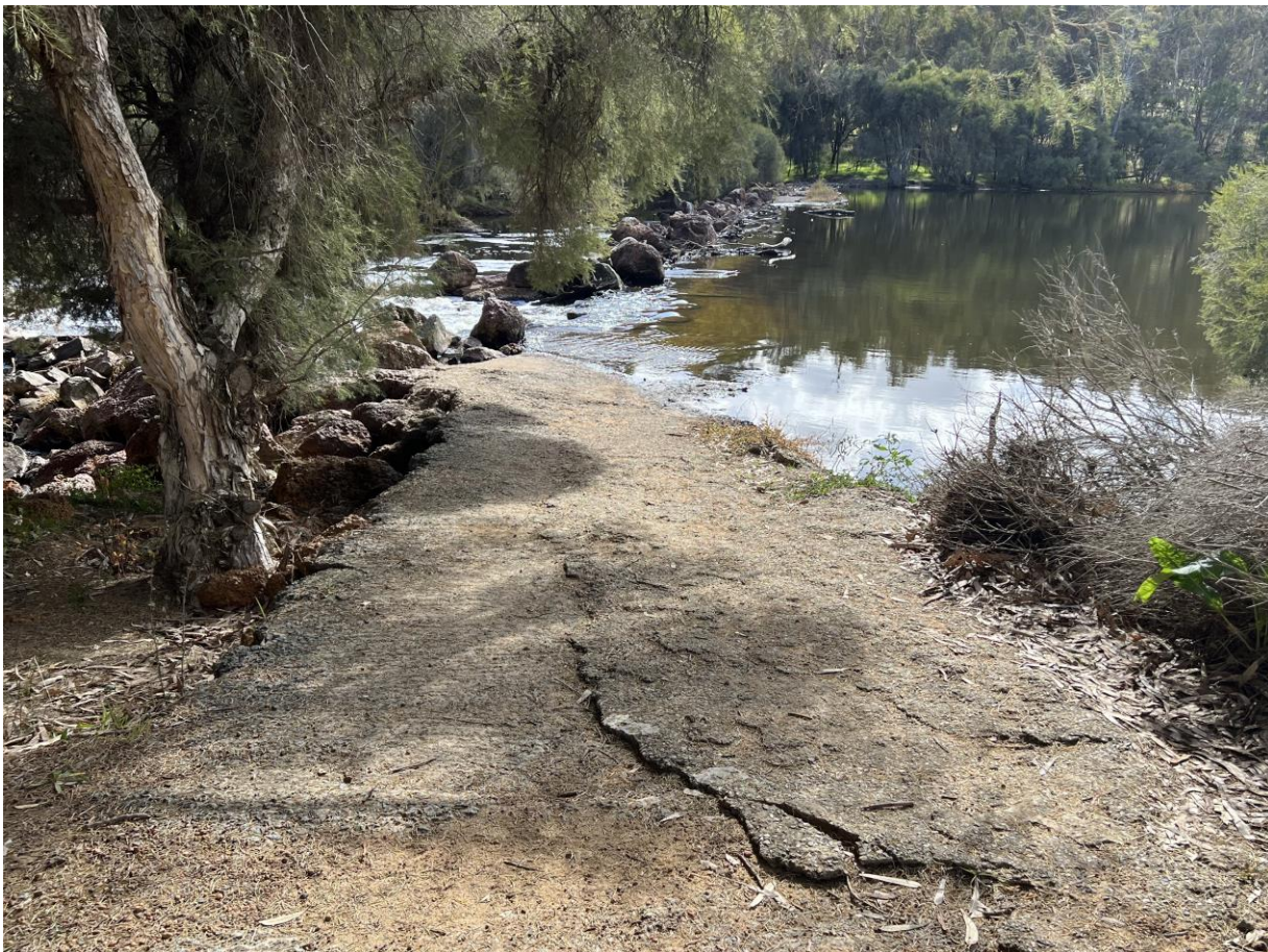
Figure 3: Photo of the Weir.
