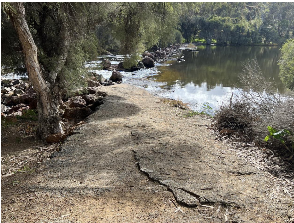
Figure 3: Photo of the Weir.
