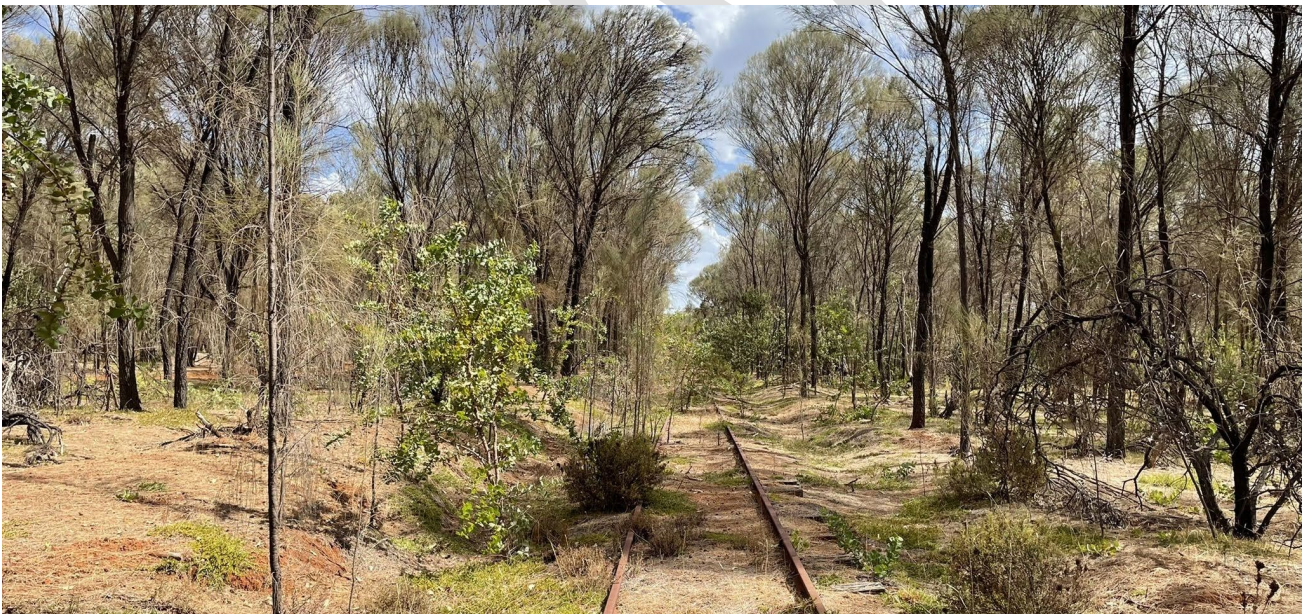
Boddington Tullis Bridge and Rail Trail
