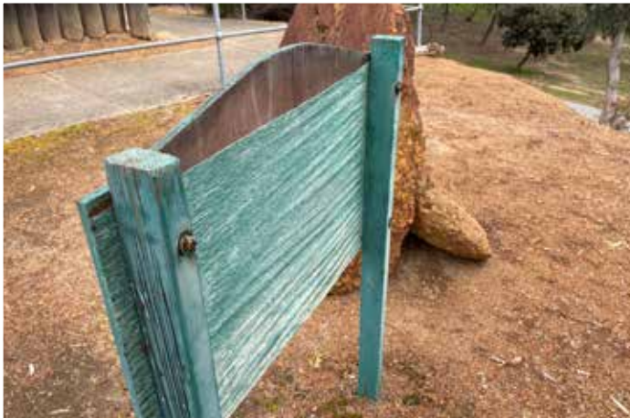
Marine ply is a poor choice of material for this type of signage.
