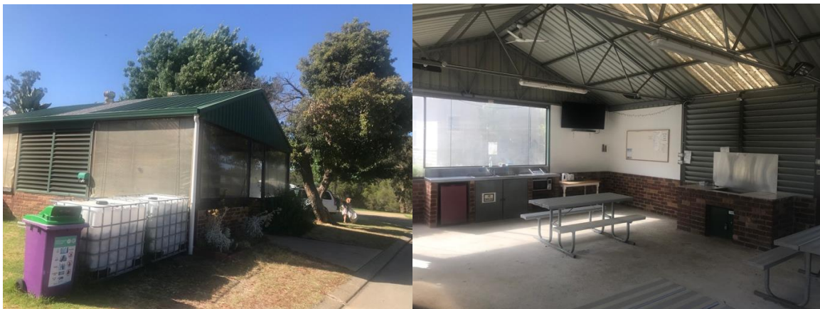
Figure 4 Existing Camp Kitchen
